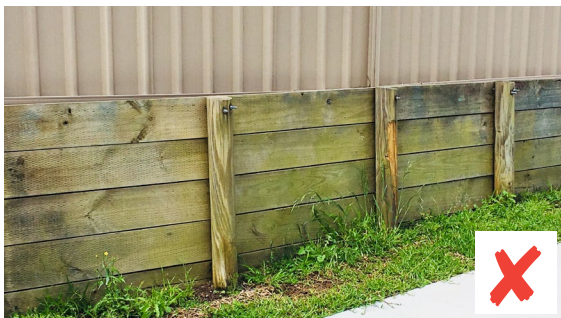
RETAINING WALLS – timber retaining walls that are visible from a public place are discouraged.
